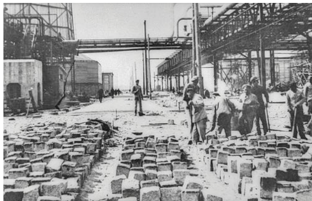
Street construction detail at IG Auschwitz, 1943-1944. USHMM WS # 79489, COURTESY OF BA
