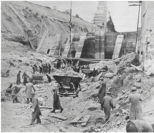
Prisoners at the Enns subcamp of Mauthausen erect a power station, nd.
