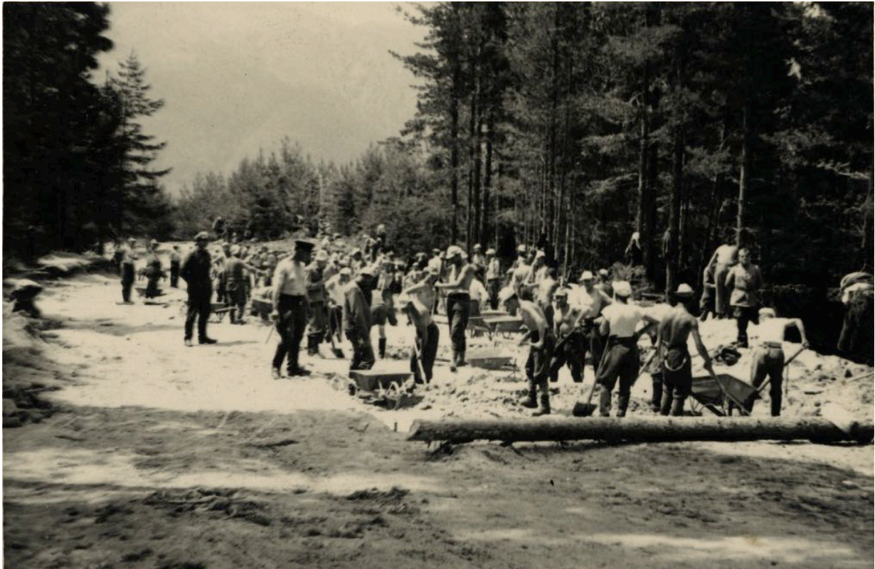
Bulgarian Jews dig a road in a forced labor brigade, 1941. USHMM WS #42245, COURTESY OF ALBERT FARHI.
