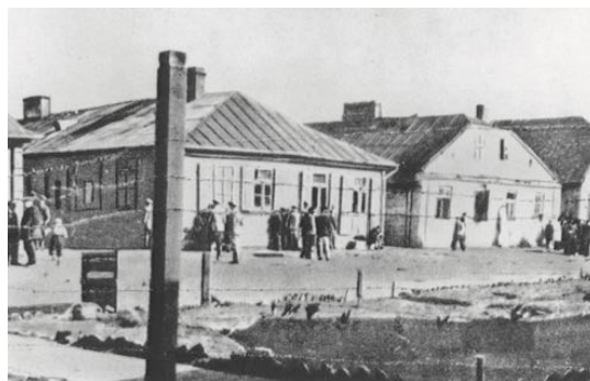
A section of the Międzyrzec Podlaski ghetto, as seen through the barbed-wire fence surrounding it, October 1942 to May 1943. USHMM WS #46319, COURTESY OF STA. HAMBURG
